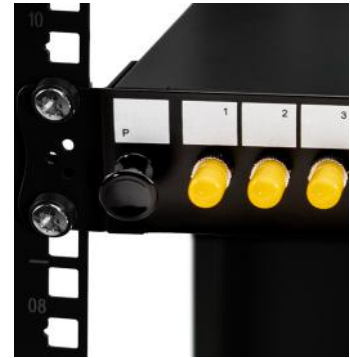
Step 4 - insert the top screws and tighten all screws
